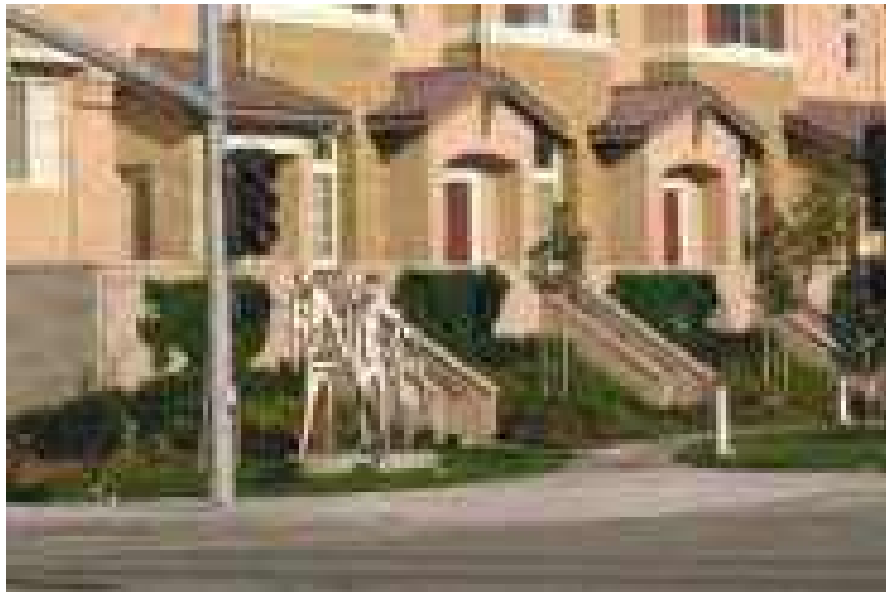
Example photos of building frontage and access.
